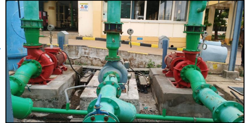
REPLACED CONDENSOR PUMPS WITH ENERGY EFFICIENT MOTORS.
